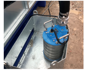
Surface mounted sump for easy maintenance
